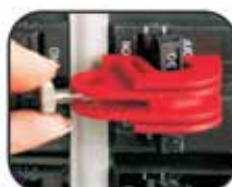
1 Tighten set screw
